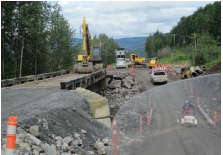
Bridge washout, Highway 97, BC
